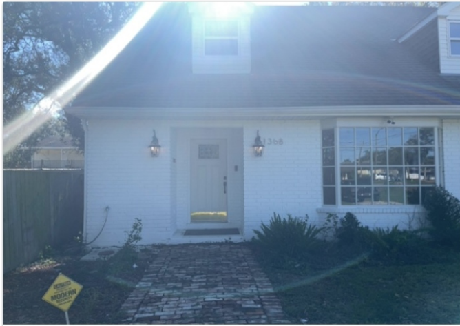
Front walkway Location: 30.020510, -90.080050 Date: Dec 15, 2022 12:15:57 PM CST
