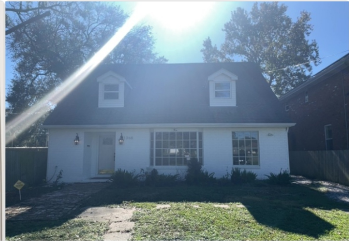
Front View Location: 30.020510, -90.080050 Date: Dec 15, 2022 12:06:47 PM CST
