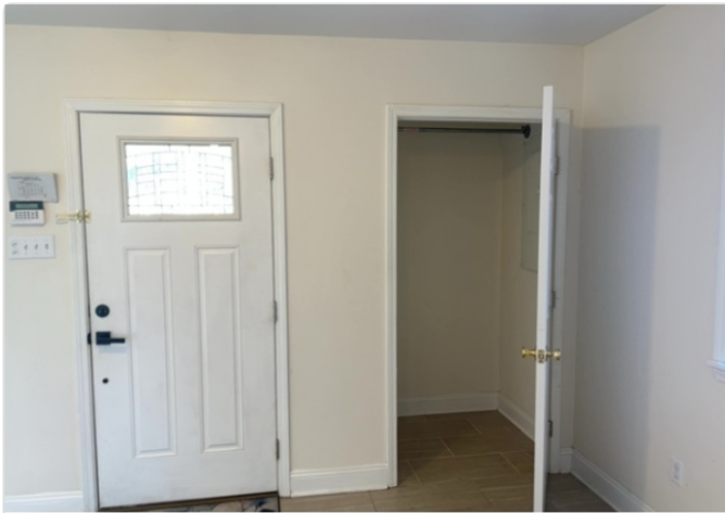
Coat Closet Location: 30.020510, -90.080050 Date: Dec 15, 2022 12:17:04 PM CST
