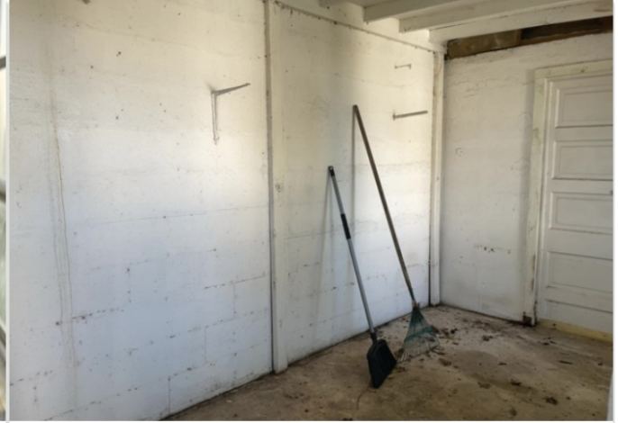
Shed Location: 30.020510, -90.080050 Date: Dec 15, 2022 12:13:12 PM CST
