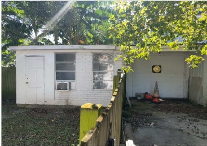
Front View Carport/Shed
