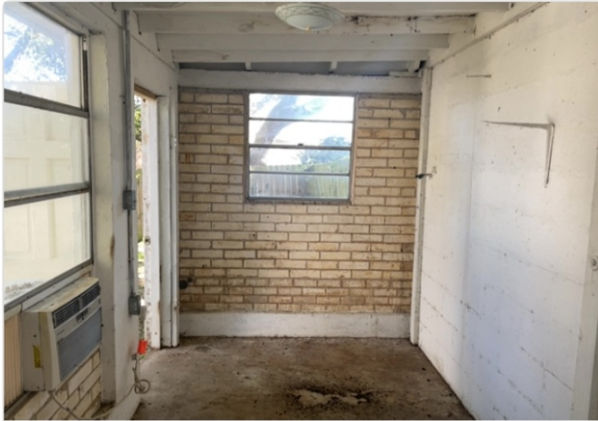
Shed Location: 30.020510, -90.080050 Date: Dec 15, 2022 12:13:25 PM CST
