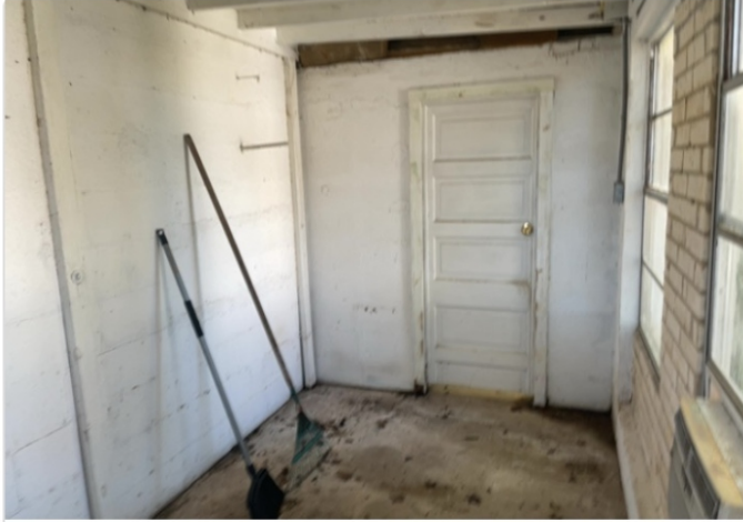
Shed Location: 30.020510, -90.080050 Date: Dec 15, 2022 12:12:59 PM CST
