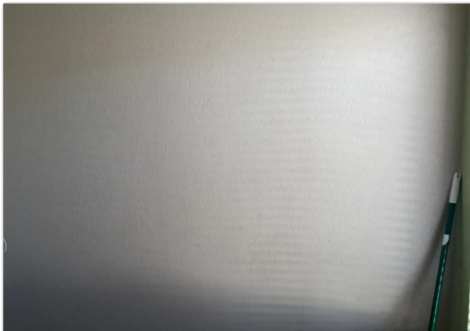
Bedroom 3 Location: 33.483427, -112.248193 Date: Feb 10, 2023 03:29:47 PM MST
