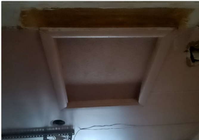
Attic Location: 33.483377, -112.248283 Date: Feb 10, 2023 03:40:13 PM MST
