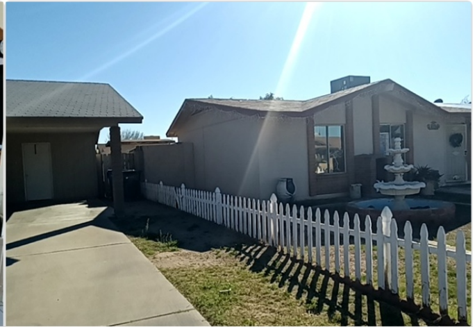
Left Side View Location: 33.483531, -112.248186 Date: Feb 10, 2023 03:04:24 PM MST
