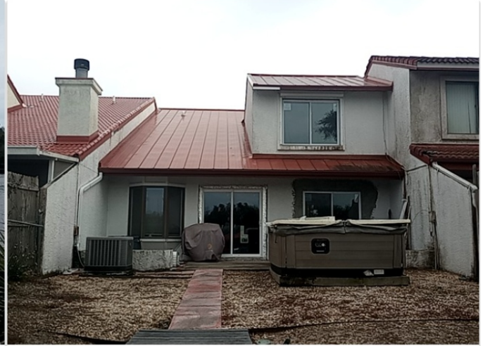
Rear View Location: 30.142163, -85.564099 Date: Dec 21, 2023 03:13:39 PM CST
