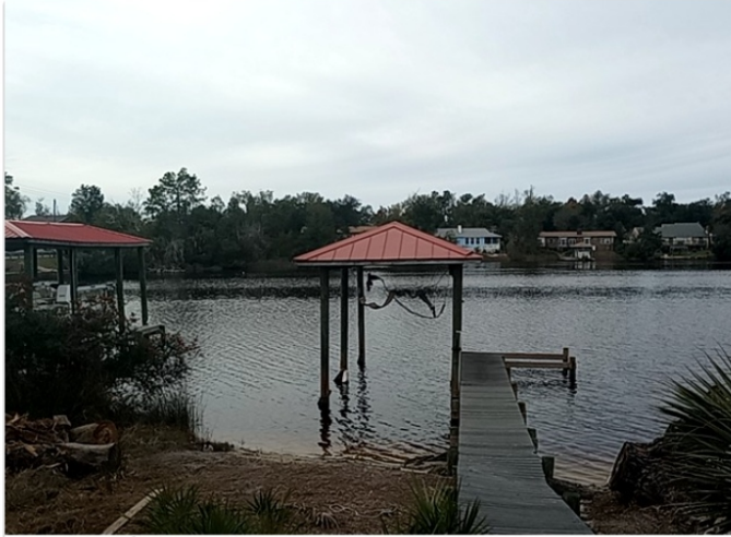
Boathouse Roof Location: 30.142163, -85.564099 Date: Dec 21, 2023 03:13:49 PM CST
