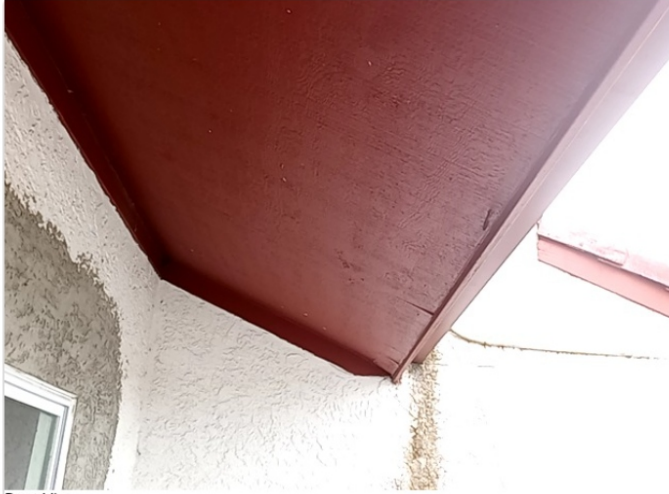
Rear View Location: 30.142163, -85.564099 Date: Dec 21, 2023 03:26:11 PM CST
