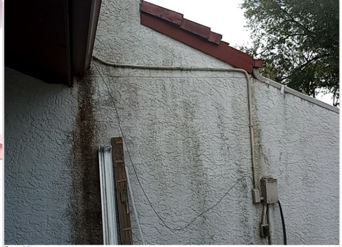
Rear View Location: 30.142163, -85.564099 Date: Dec 21, 2023 03:26:25 PM CST
