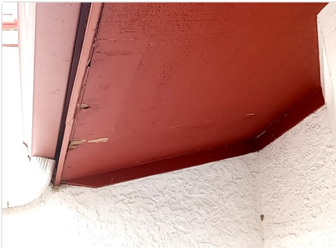
Rear View Location: 30.142163, -85.564099 Date: Dec 21, 2023 03:25:41 PM CST
