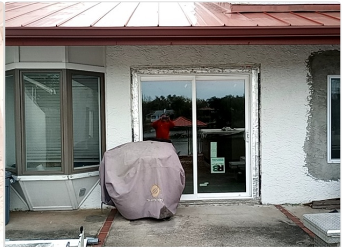
Rear View Location: 30.142163, -85.564099 Date: Dec 21, 2023 03:25:58 PM CST
