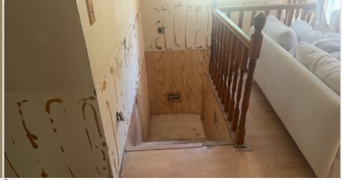
Stairs Location: 34.237461, -117.280504 Date: Oct 16, 2023 11:44:46 AM PST
