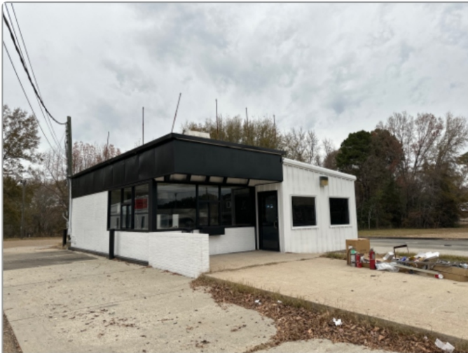
Exterior Photo - Left Side View
