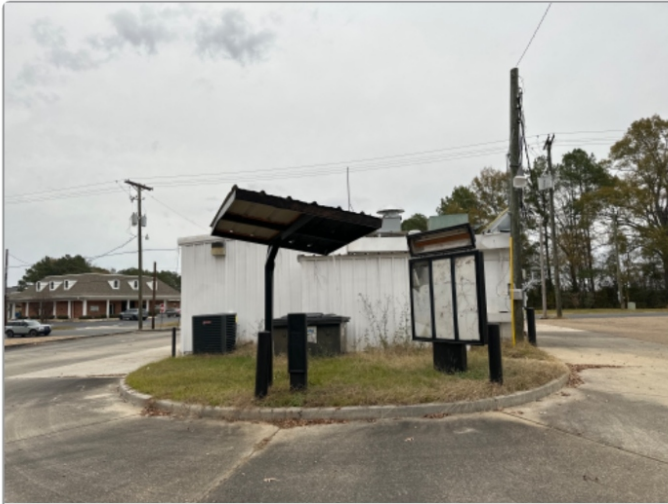
Exterior Photo - Entire Back View
