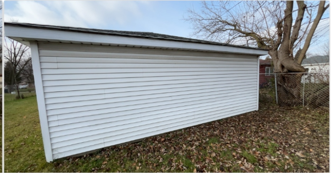
Rear View Garage Location: 41.594539, -87.657991 Date: Dec 06, 2023 12:12:42 PM CST
