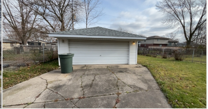
Front View Garage Location: 41.594539, -87.657991 Date: Dec 06, 2023 12:12:09 PM CST
