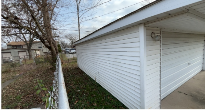
Left View Garage Location: 41.594539, -87.657991 Date: Dec 06, 2023 12:13:07 PM CST
