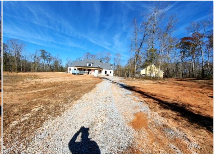
Clearing Location: 33.120075, -84.203684 Date: Nov 27, 2023 01:43:59 PM EST
