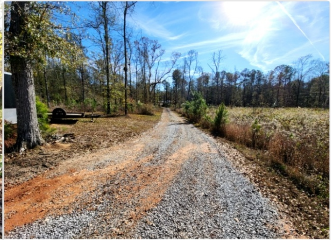
Temp driveway Location: 33.120075, -84.203684 Date: Nov 27, 2023 01:43:31 PM EST
