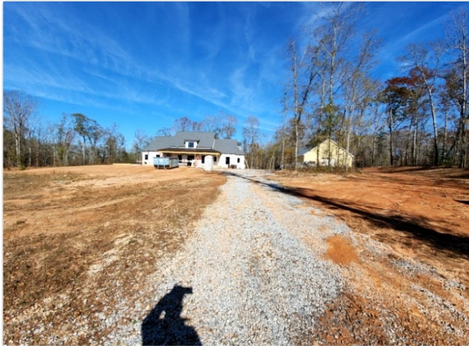
Temp driveway Location: 33.120075, -84.203684 Date: Nov 27, 2023 01:43:40 PM EST
